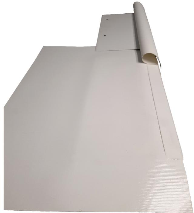
3. Align the Duro-Edge to within 1/4 inch of the parapet wall edge. Press the Duro-Edge firmly into the approved Duro-Last sealants to set its position.
