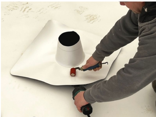
Figure 7 (Weld Stack Flashing)
