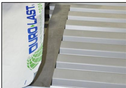
4. On steel decks, at the end of a roll, install a metal plate (6 in. by 42 in.) to support the vapor barrier end lap between the metal flutes ensuring a complete end lap seal. End laps must overlap by 6 inches.
