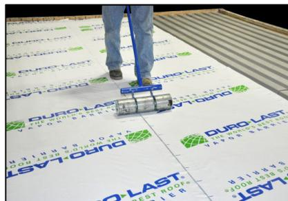
3. Install subsequent rolls of vapor barrier in the same way, taking care to overlap the longitudinal joints by 3 inches.
