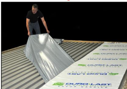
2. Once the vapor barrier is in place, while holding the product tight, peel off the silicone release film by pulling diagonally.
