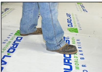
5. The vapor barrier offers extra protection from heavy foot traffic during installation. The slip-resistant surface allows for safe movement across the roof.
