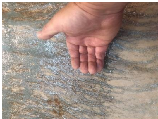
Checking for dry Solvent-Grip Plus
